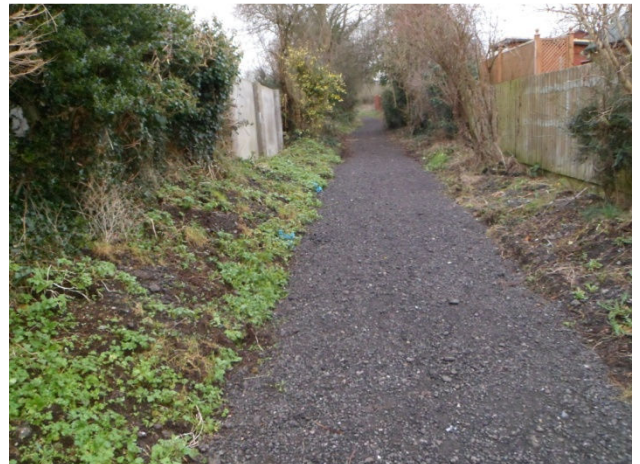
Byway 89 After Surfacing
